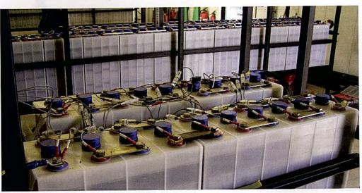
The programme to upgrade the DC backup power systems at the compressor stations is focussing on three main types of battery systems: fire and gas detection; switchgear control; emergency power. The first two systems are supported by 24V batteries, while a 110V battery provides the emergency power.
